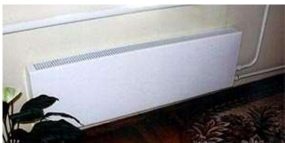
**Steel panel radiator** is a rectangular panel consisting of two welded together steel sheets with extruded flutes forming channels for circulation of heat transfer mediums. Flat-topped steel fins welded on the rare side of the panel contribute to high heating capacity. A number of such panels
